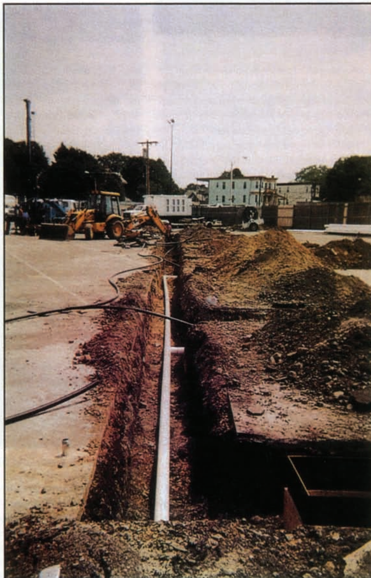
Remedial wall installation.
